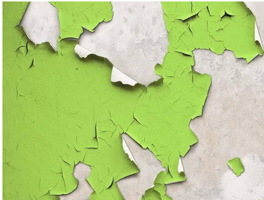
Figure 19 Intercoat Peeling
