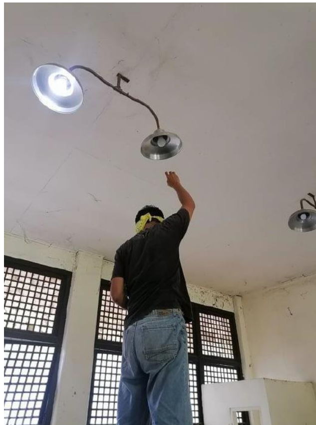
Figure 34 Replacing Incandescent Bulb
