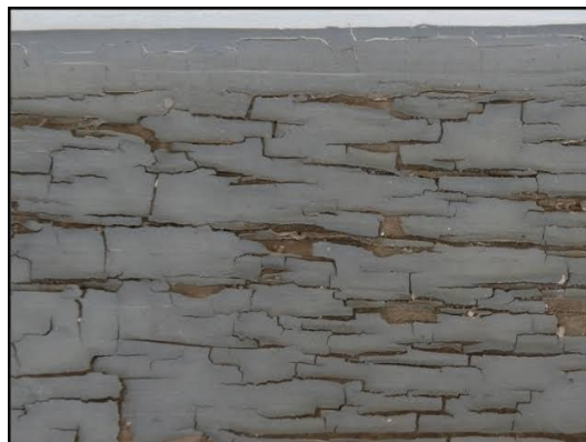
Figure 20 Cross-grain Crackling
